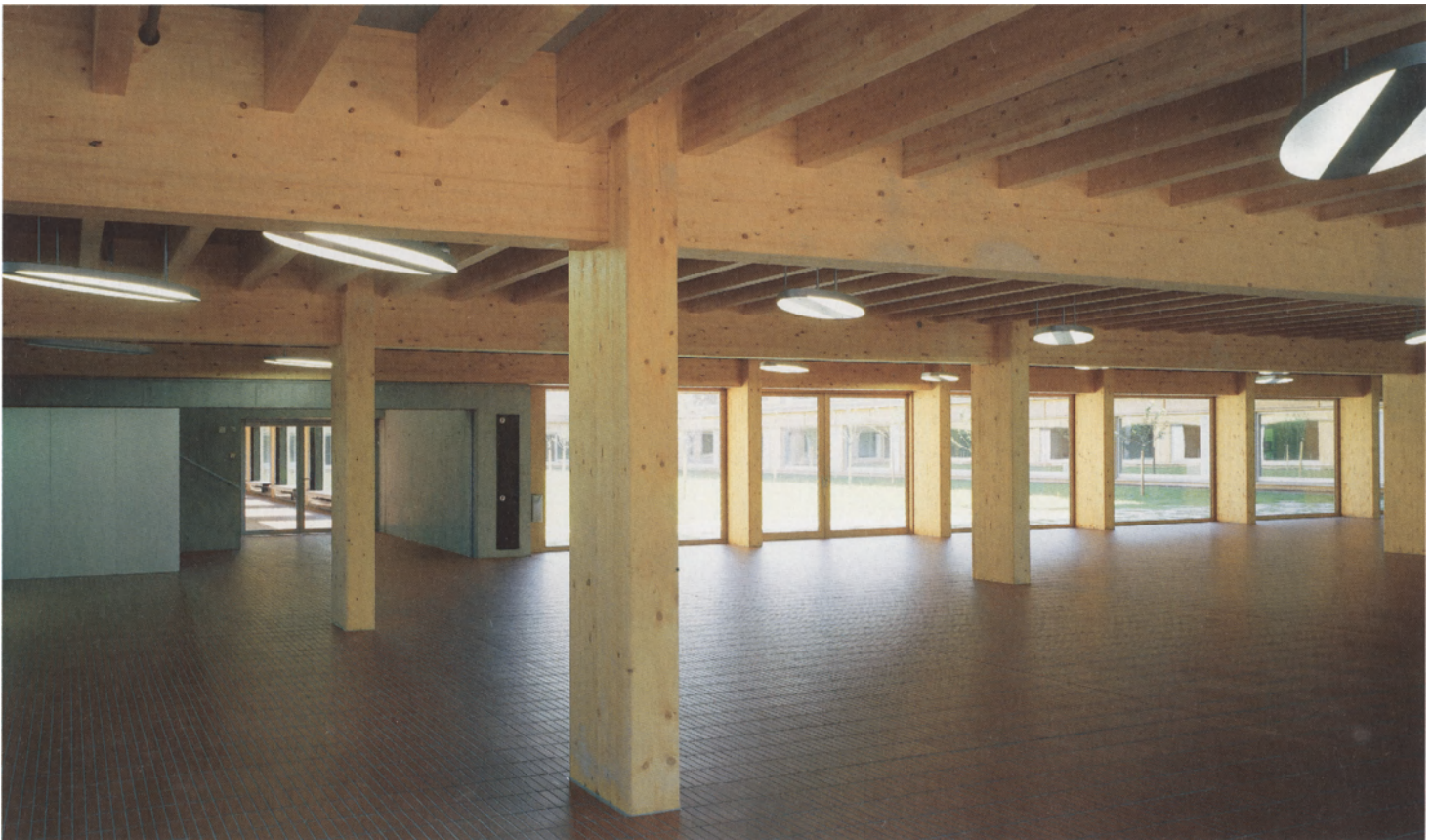
b125 Loadbearing structure in frame construction, school, Wil, Switzerland,
