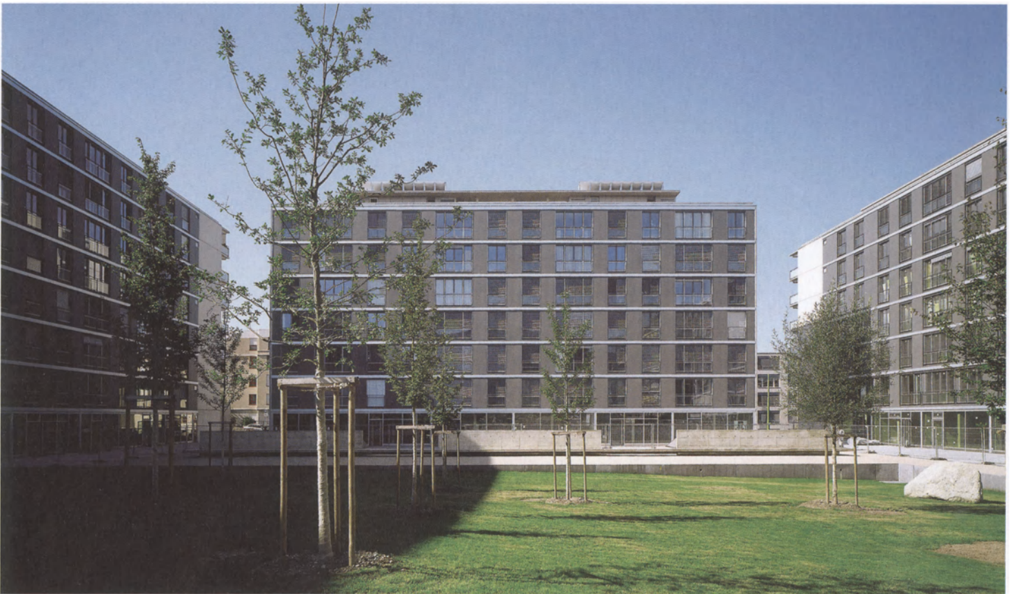
b28 An example of the combination of different materials: eight-storey apartment block, Grand-Saconnex, Geneva, Switzerland; loadbearing construction in reinforced concrete, facade elements in timber, incombustible facade cladding (for sketch of this principle see Fig. b30)
