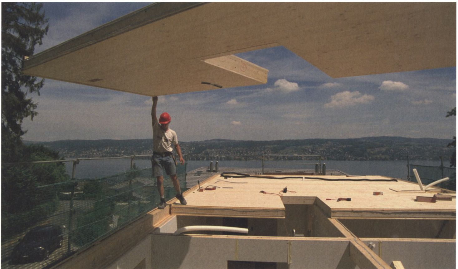
b116 Erecting hollow-box floors for a timber building in panel construction
